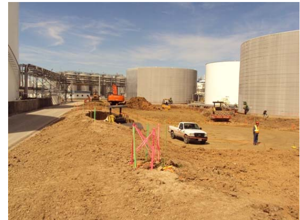
Start up for expansion construction in Houston
