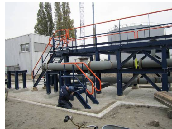
New manifold for OTR pipeline project
