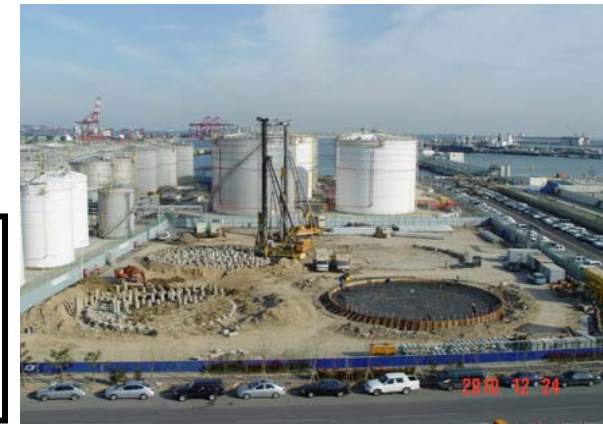
OTK expansion underway
