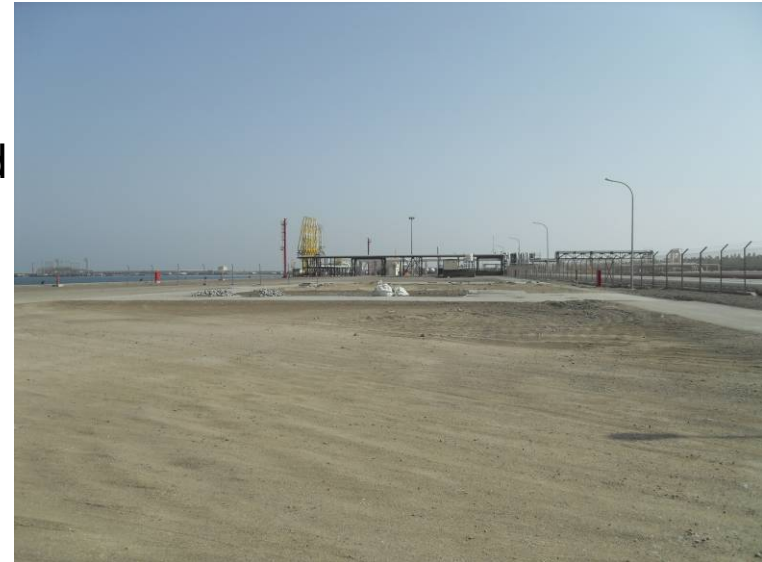
The expansion area for chemical storage at OOT
