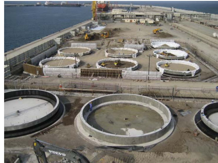
Construction new tanks at OOT, Sohar
