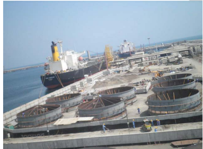
New OOTO tanks under construction (Sept. 2011)
